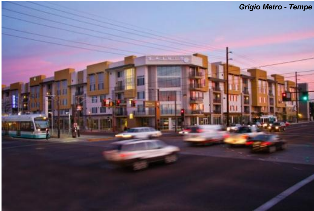
Figure 5-1. Example of Transit-Oriented Development in Tempe, AZ
